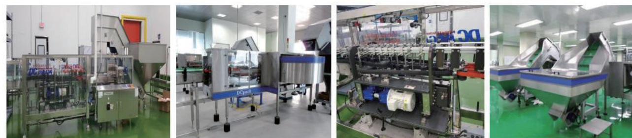
実際の現場設置姿 / Installed at site
